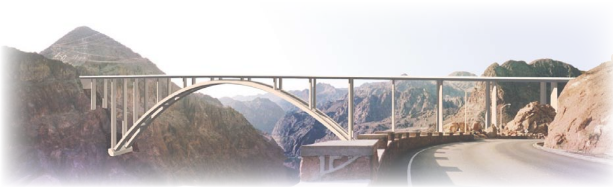
Photo of Hoover Dam Bypass Project Photo credit: www.hooverdambypass.org
